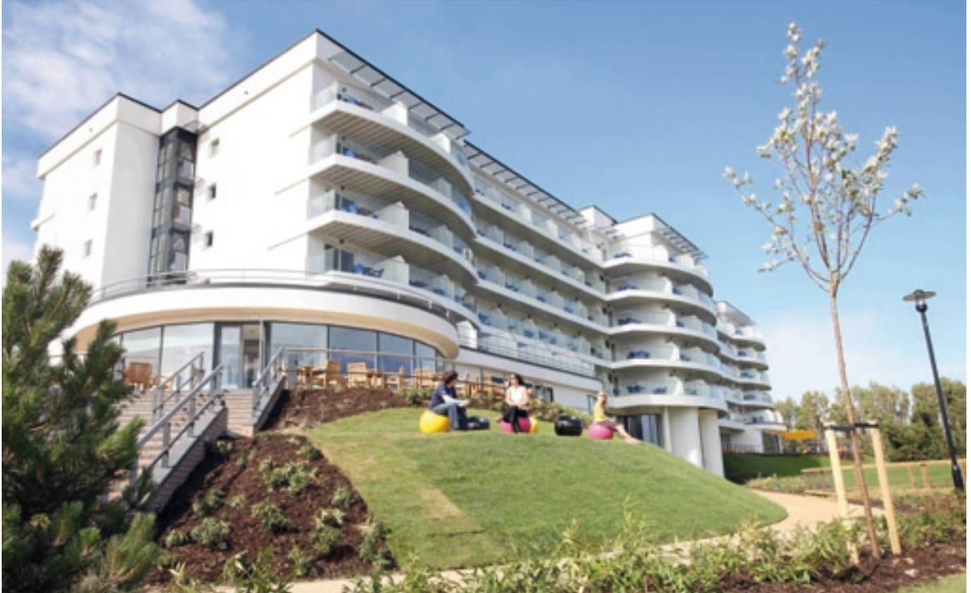
Composite curtain walling system REHAU Polytec 50S combines the benefits of Aluminium, Steel and Polymer materials providing an outstanding thermal performance with an  $U_f$ -Value of up to  $0.88 \text{ W/m}^2\text{K}$ .
