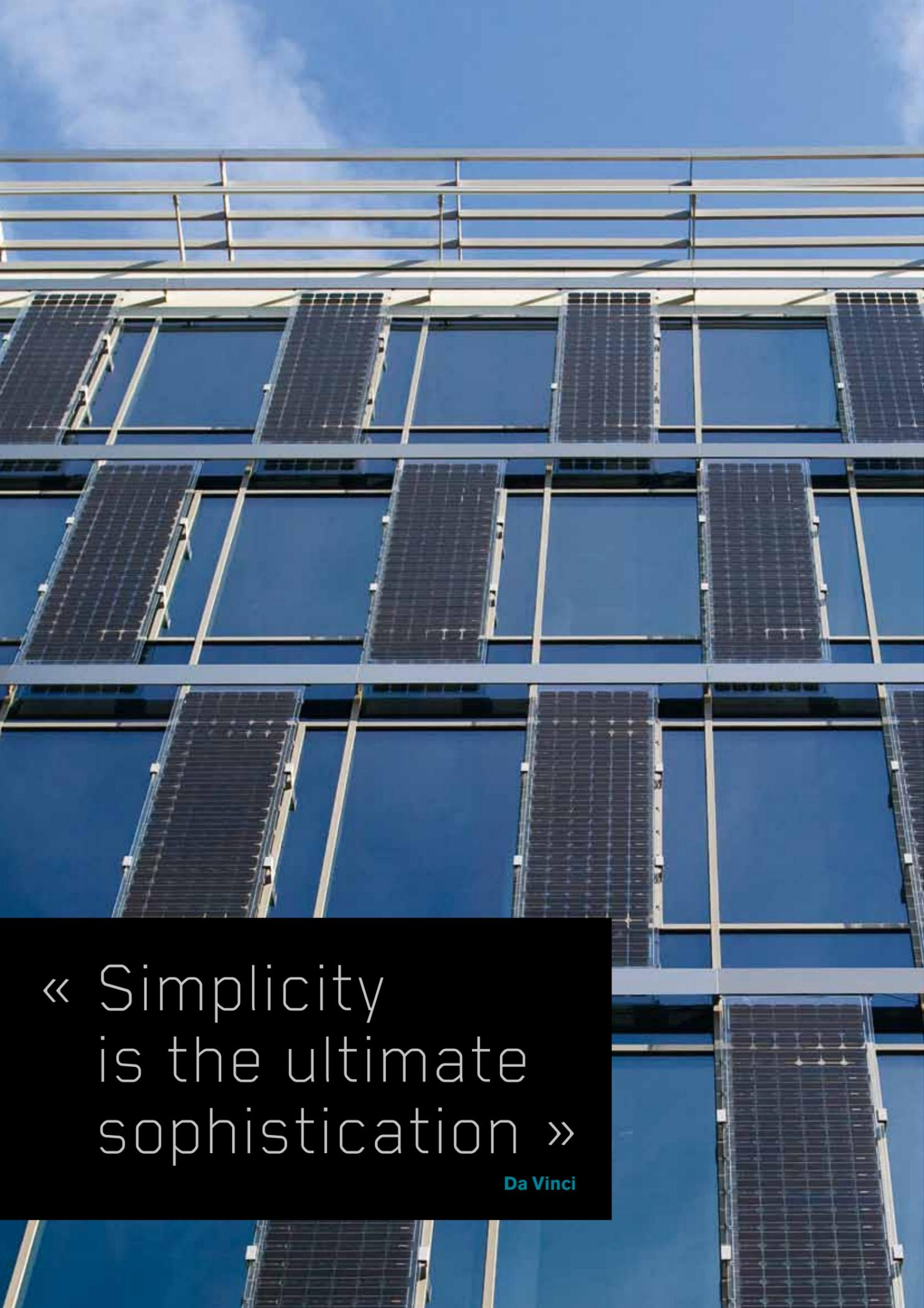
NRGY 62 is an innovative facade system that combines smart profile design with the demands of contemporary building design. It allows large glass sizes to maximize light penetration.
